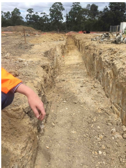
Figures 1a and 1b. Dense clay subsoils excavated for tree pits. Note the smearing of the clay (right) by the excavator bucket.
