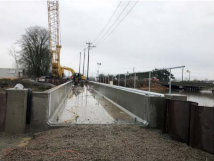
Photo 2 – Bridge Deck Complete Pre-Ballasting
