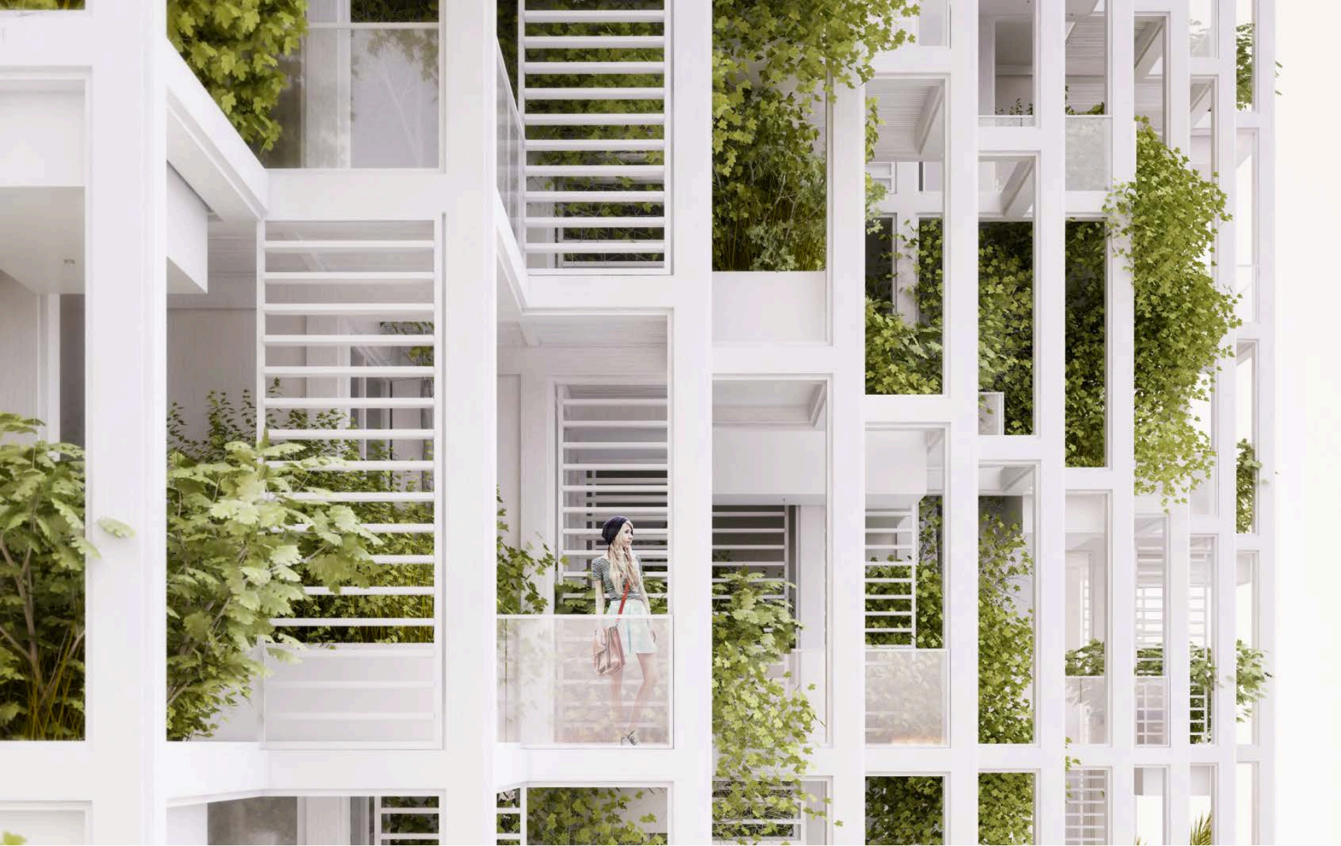
Vijayawada Garden Estate, India Penda Architects
