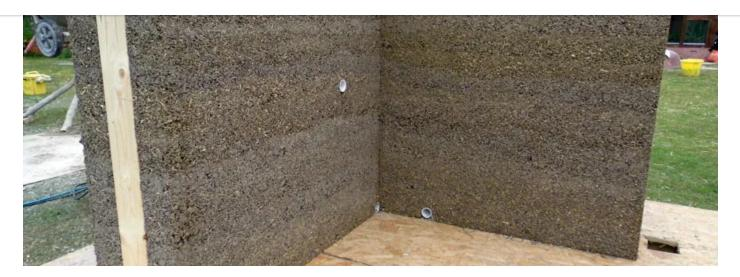
Perhaps the most definitive feature of Hempcrete is its resilience to common problems faced by building materials. Hempcrete is highly flame-resistant; this lends buildings constructed with Hempcrete an inherent fire-proofing that is built into the very walls of the structure. Further, as it uses a lime binder, Hempcrete is extremely resistant to fungus, and also has anti-microbial properties. This means that Hempcrete can resist the formation of mold in even highly humid conditions.
