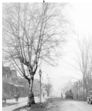
1917 First Street Tree bylaw established protection, and assigns care and custody to the Vancouver Park Board
