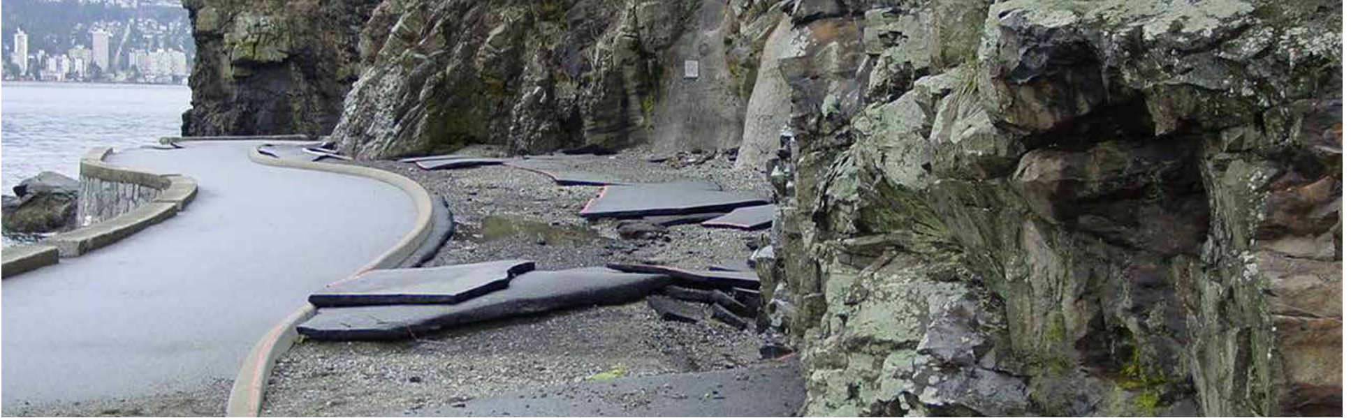
Stanley Park seawall damage, 2012
