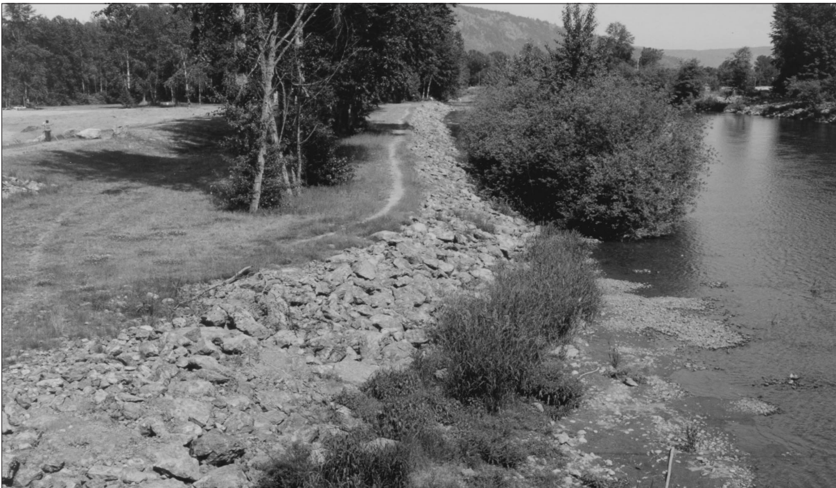
Bank protection and riparian vegetation – Cowichan River
