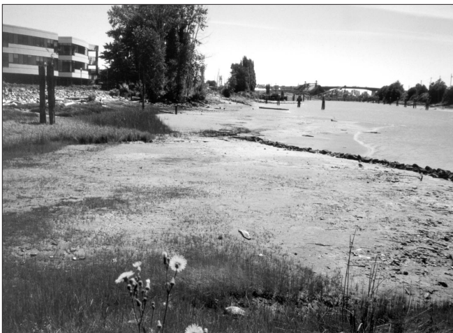
Healthy Habitat and dike structures can co-exist – Lower Fraser River
