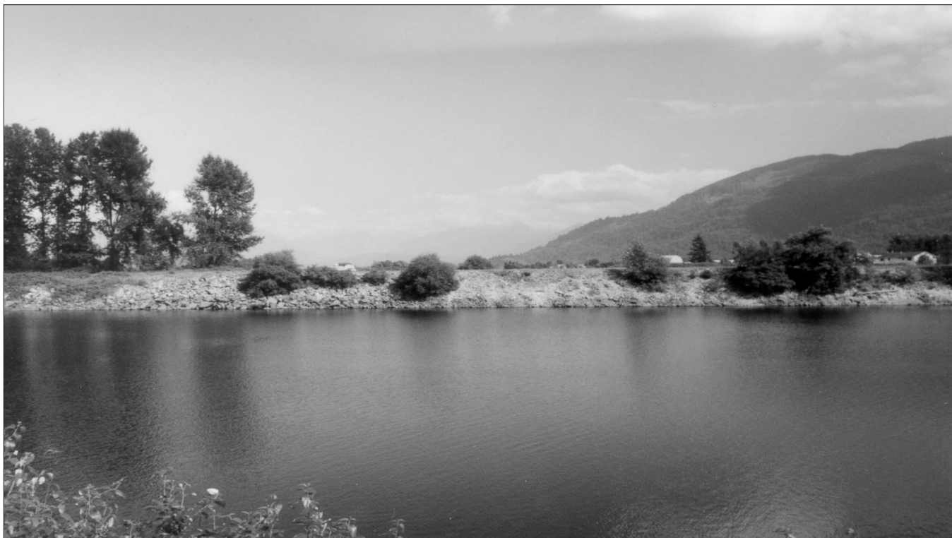
Riverside dike with bank protection and acceptable vegetation clumps.
