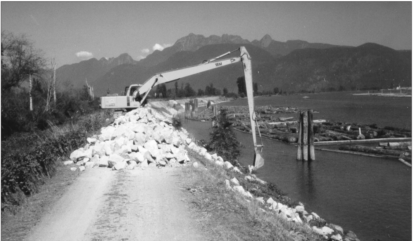
Preserving a vegetation clump while repairing bank protection – Pitt River
