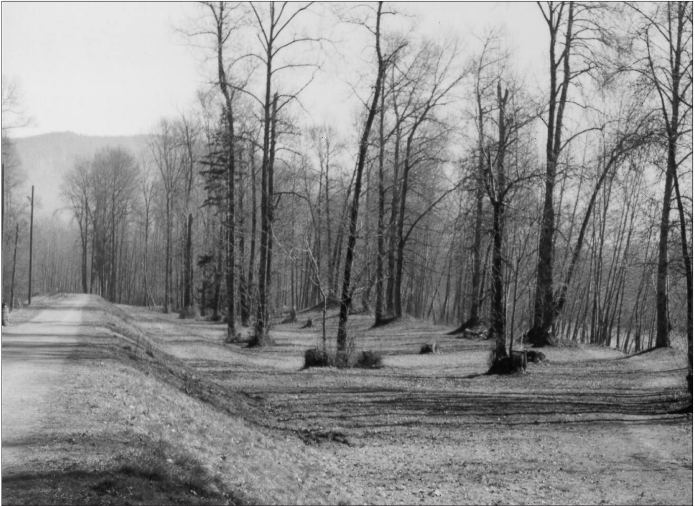
Setback dike with riparian vegetation preserved on overbank – Cowichan River
