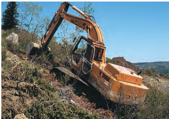
Topsoil salvage prior to construction.
