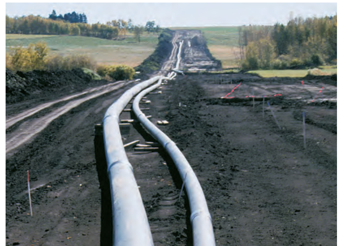
A pipeline in the Parkland Region of Alberta.
