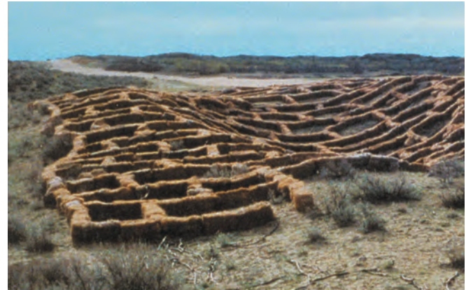
Straw bales are laid out in cell patterns to reduce wind erosion on sandy soils.
