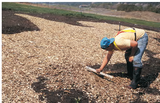
Spreading clean aspen chips on a revegetation site.
