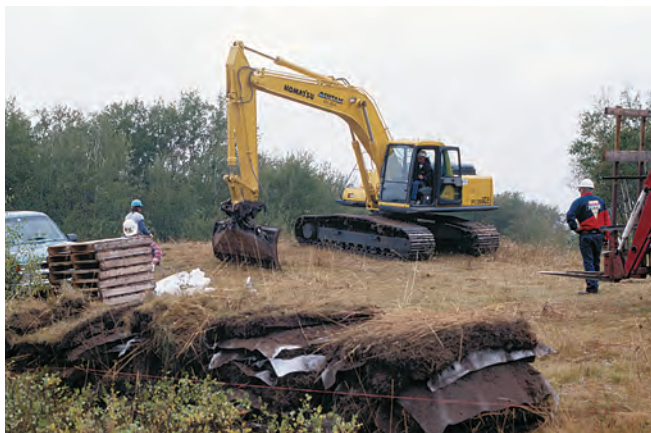
A concrete cutting blade is mounted on the front blade to cut sod.
