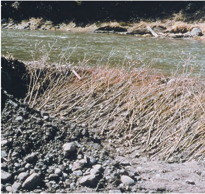
Bundles of willow whips are placed along banks – as they grow they will stabilize the bank.
