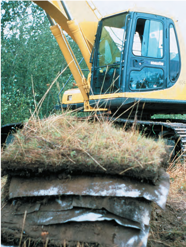
Salvaging sod during pipeline construction in the parkland area of Alberta.
