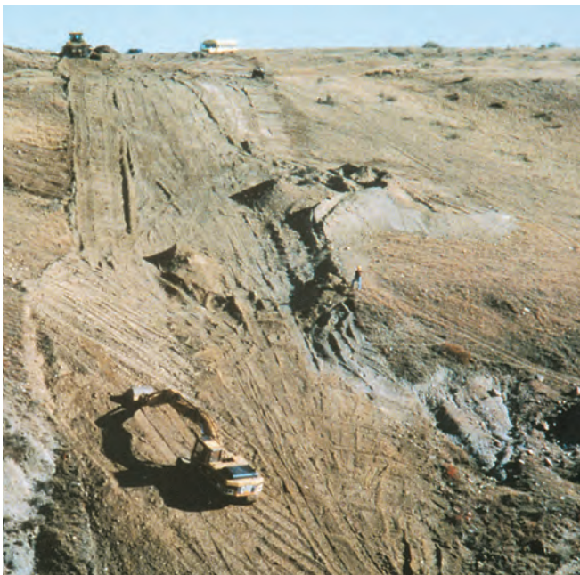
Erosion control is a primary concern on steep slopes.
