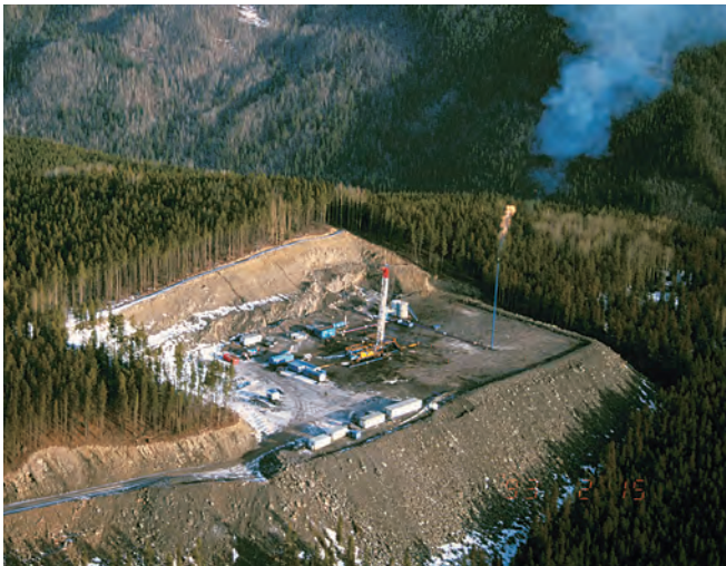
Wellsite in the Rocky Mountains.
