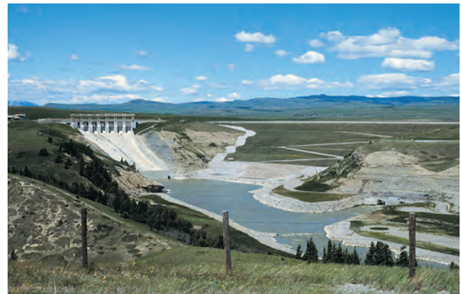
Oldman River Dam.
