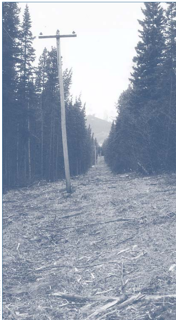
PHOTO: ATCO ELECTRIC
