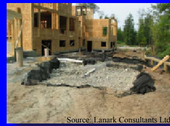
Source: Lanark Consultants Ltd
