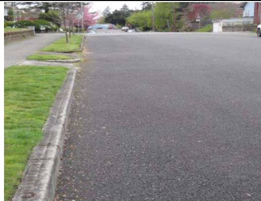
Porous asphalt installed curb to curb on a residential street (Source: City of Portland, Bureau of Environmental Services)
