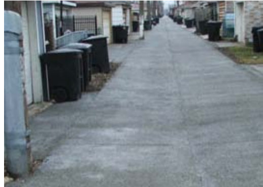
PerVIOUS concrete applied to an alleyway in Chicago (Source: City of Chicago)
