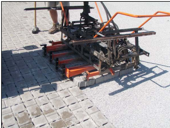
Permeable pavers being mechanically placed in sections (Source: CVC)
