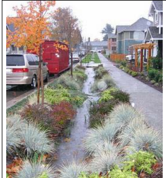
Figure 3.2.6. Open drainage applied in a medium density neighbourhood
