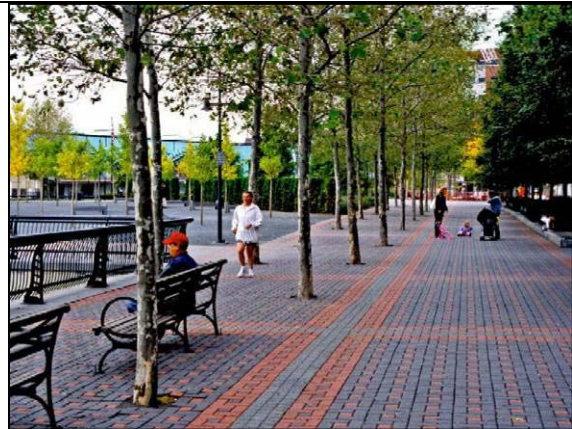
Permeable pavers in Hoboken, NJ used around trees which allow air and water to reach the roots (Source: Bruce Ferguson).
