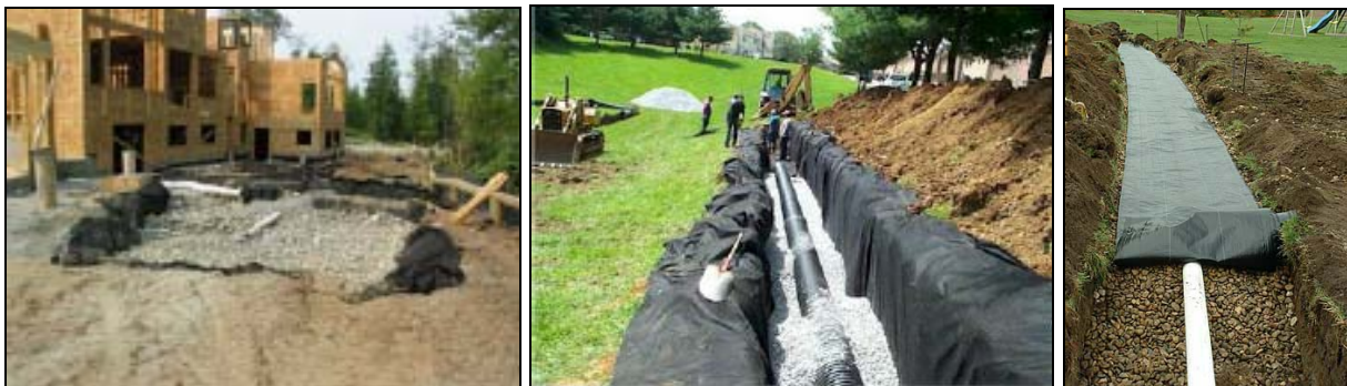
Figure 4.4.1 Construction of a soakaway in a residential subdivision and infiltration trenches in parkland settings
