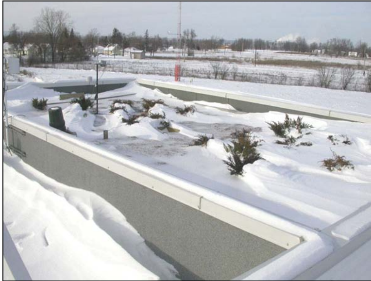
Figure 4.2.2 A green roof during winter
