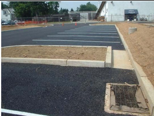
Porous asphalt parking lot (Source: Villanova Urban Stormwater Partnership)
