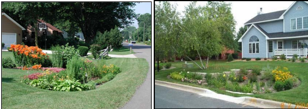
Left and Right - front yard rain gardens that takes runoff from the residential lot and street (Source: City of Maplewood, Minnesota)
