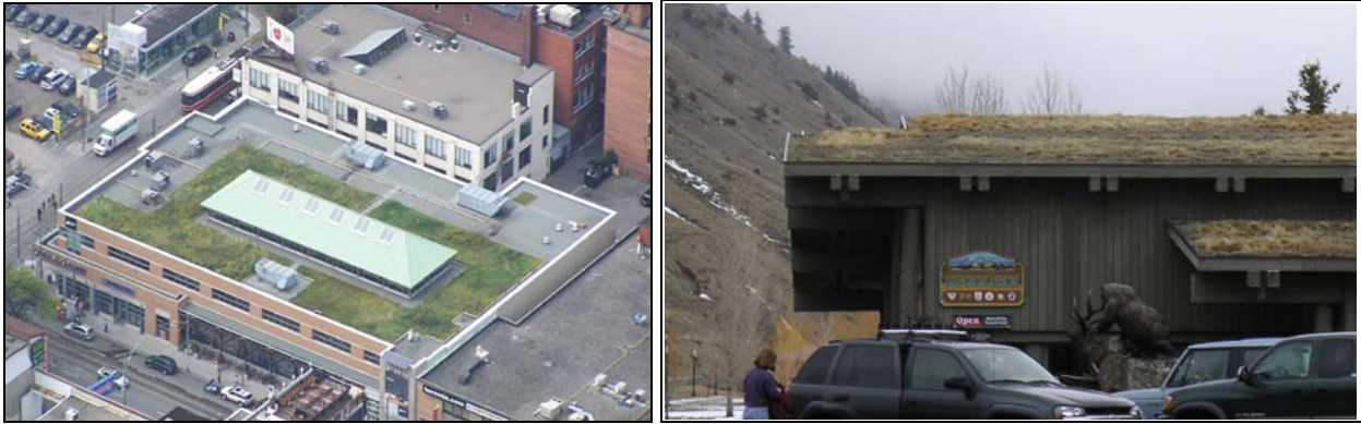
Source: City of Toronto (left); CWP (right)
