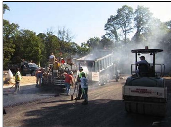
Porous asphalt installation (Source: Villanova Urban Stormwater Partnership)
