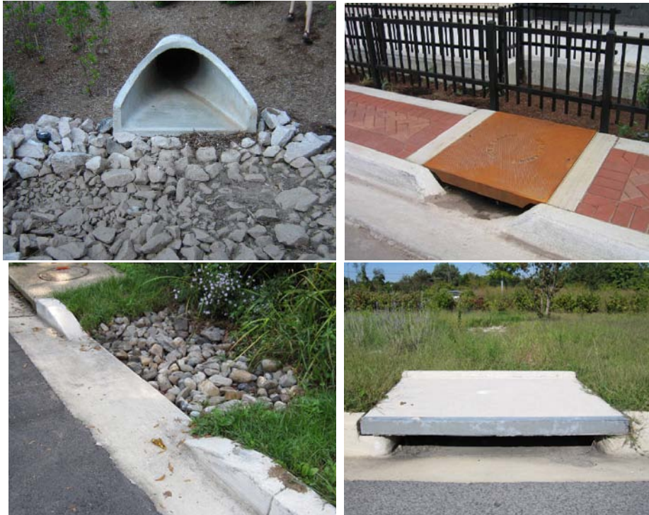
Figure 4.5.10 Examples of inlets to bioretention practices
