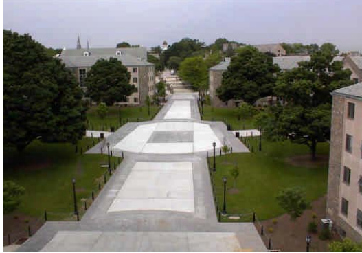
PerVIOUS concrete walkway plaza (Source: Villanova Urban Stormwater Partnership)
