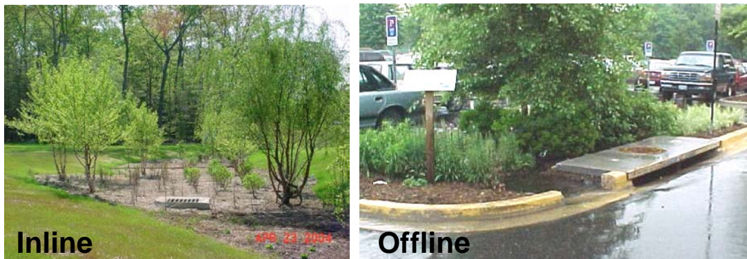
Figure 4.5.9 Examples of inline and offline bioretention
