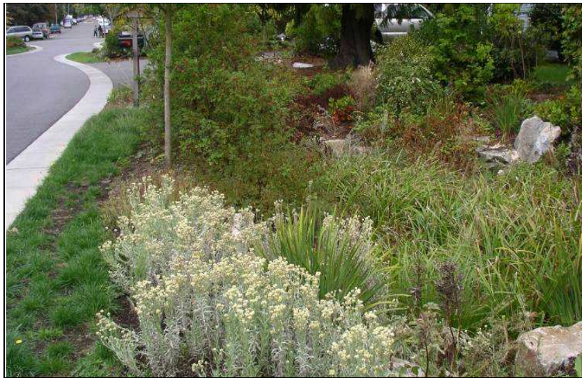
Figure 31 – Dry swale constructed as part of the Seattle Public Utilities Street Edge Alternative program. (Source: Center for Watershed Protection)
