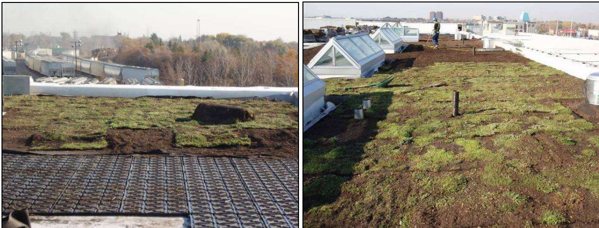
Figure 7 – GO Transit bus facility extensive green roof installation with pre-grown mats, Mississauga, ON (Source: CVC)
