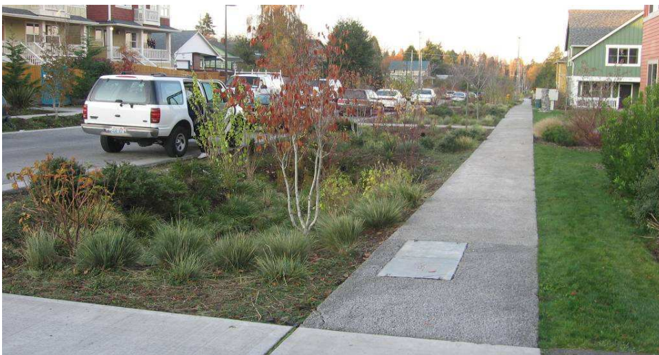
Figure 32 – Dry swale planted with a mix of herbaceous, shrub, and small trees in Seattle, WA (Source: CVC)
