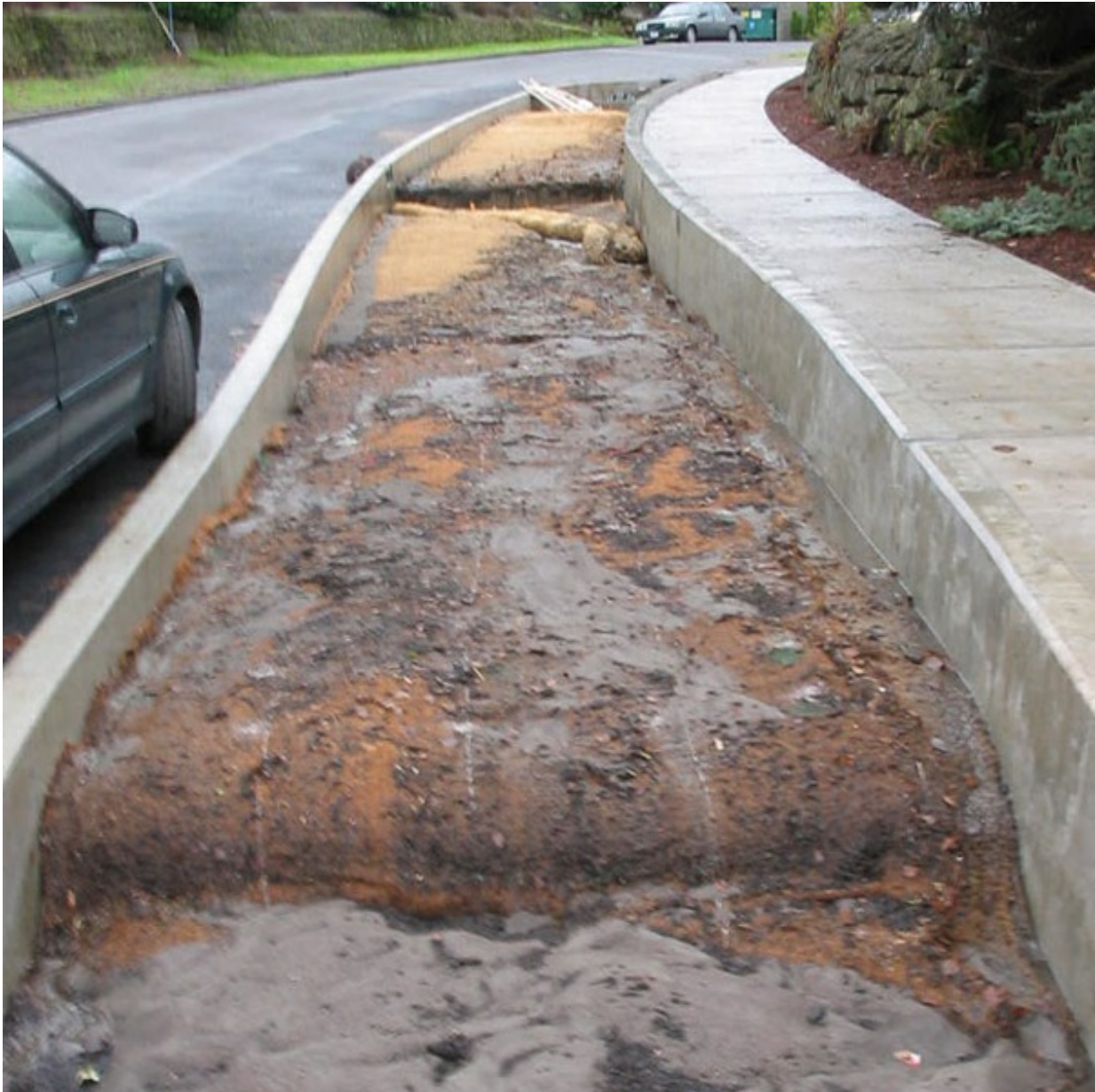
Soil erosion and displacement in an unplanted bioretention planter. / image: City of Portland
