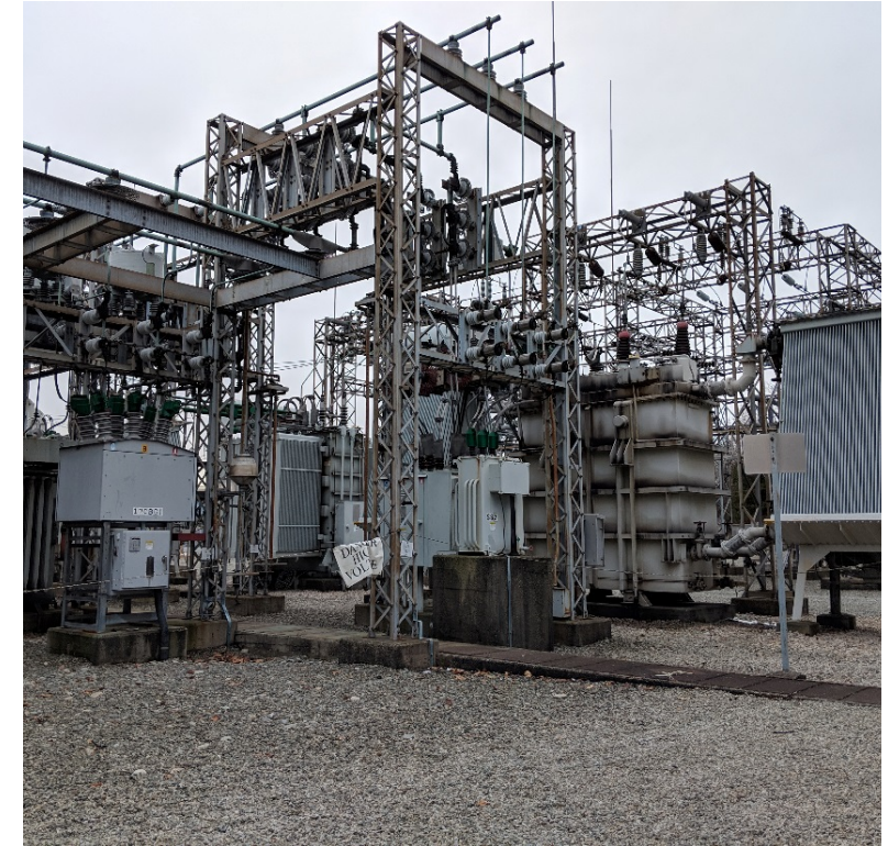
A substation in the floodplain
