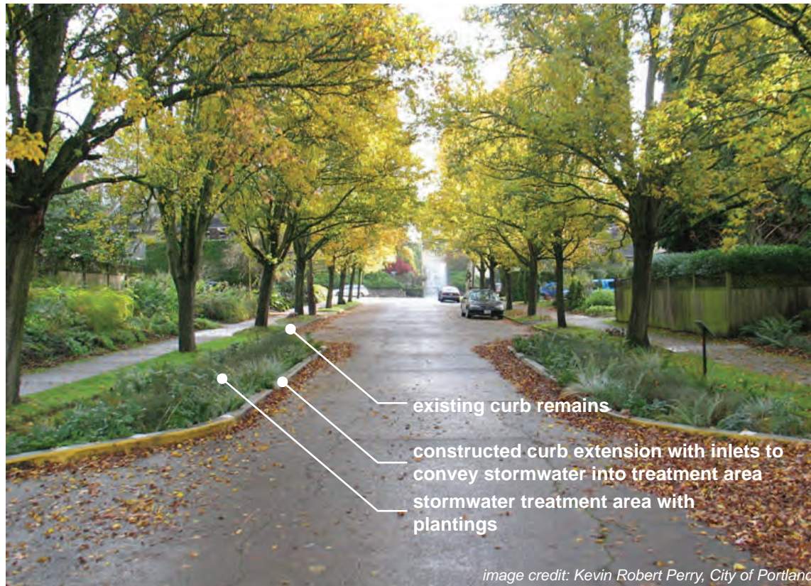
Figure 7: A LID Street Stormwater Retrofit - Siskiyou Street, Portland, Oregon
