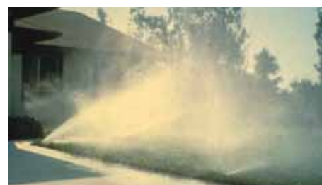
Far Left: Online landscape scheduling calculator. Above Right: Automated irrigation system. Above: Irrigation system operating at excessive pressure.
