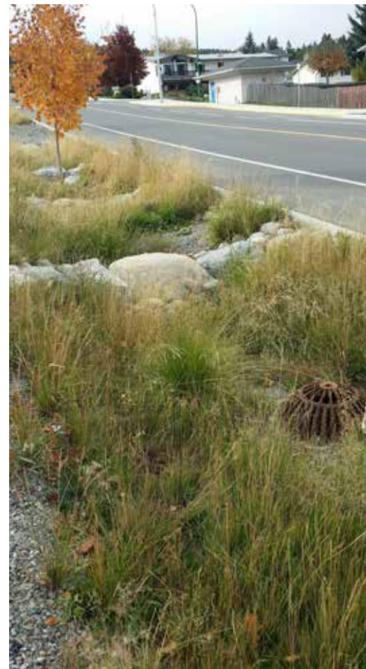
Figure 1. One of our “naturalized” bioswales working hard and waiting to be loved. Photo credit: Shasta McCoy
