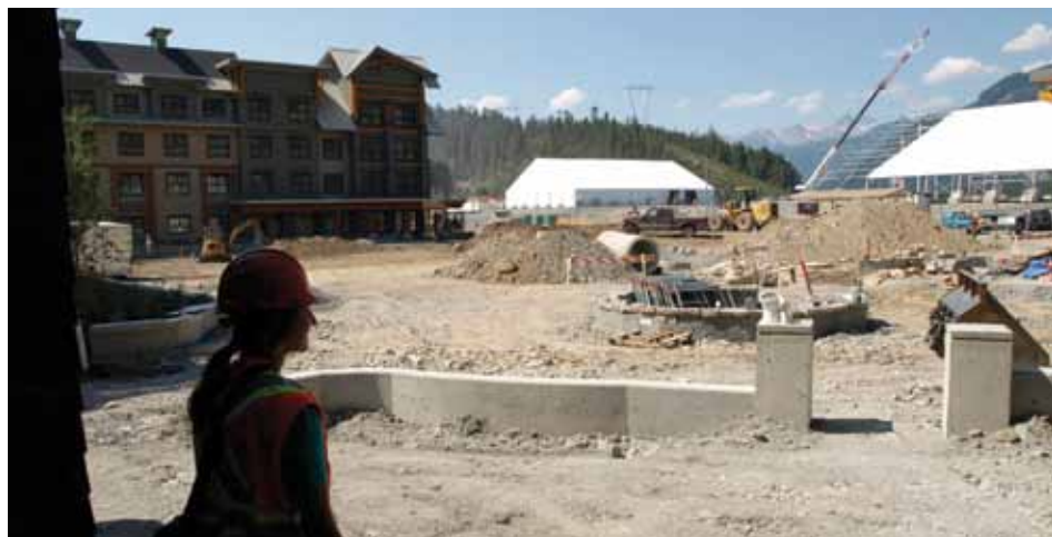
Construction of Whistler Athlete Commons Park – 2009. Image courtesy of Tom Barratt Ltd.
