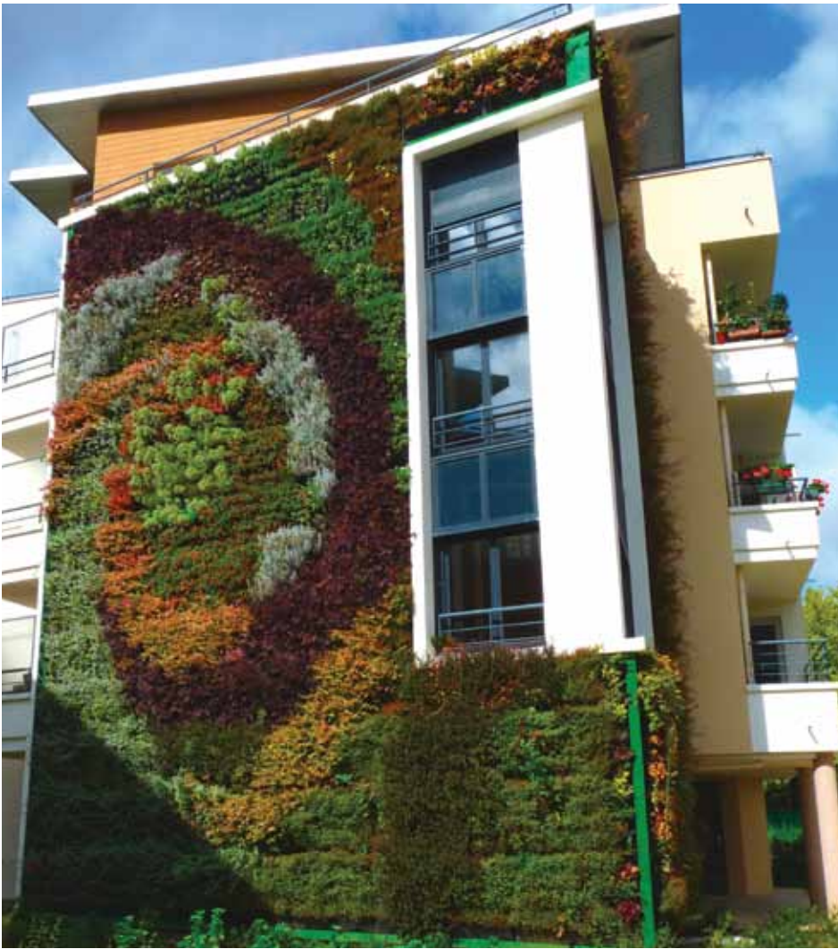
ModuloGreen exterior living wall. Image courtesy of Nicolas Rousseau.
