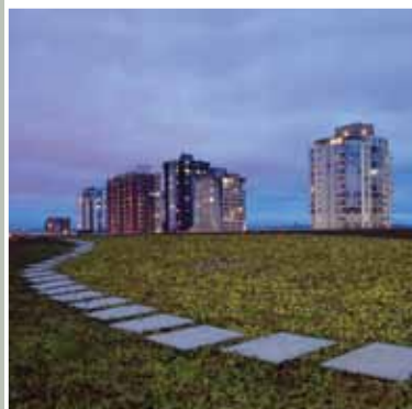
Cover Image: Local green roof supplied and installed by Architek. Image courtesy of Ron Schwenger.
