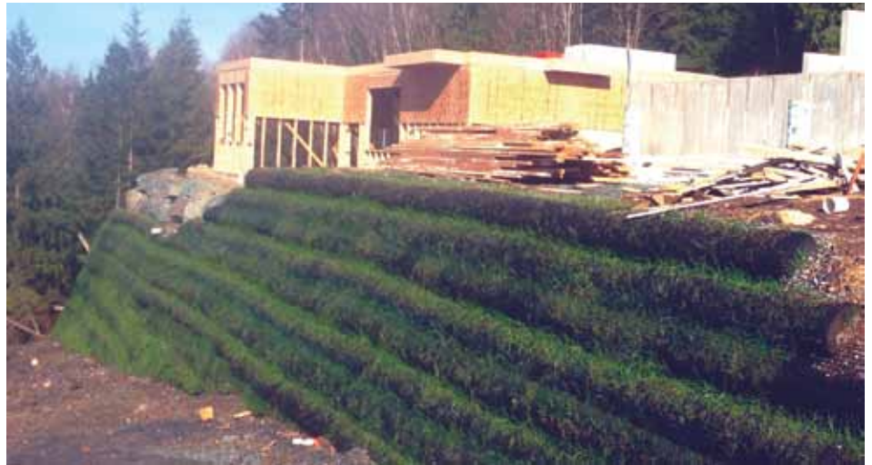
Cascade Live Retaining Wall by Denbow. Image courtesy of David Adkins.
