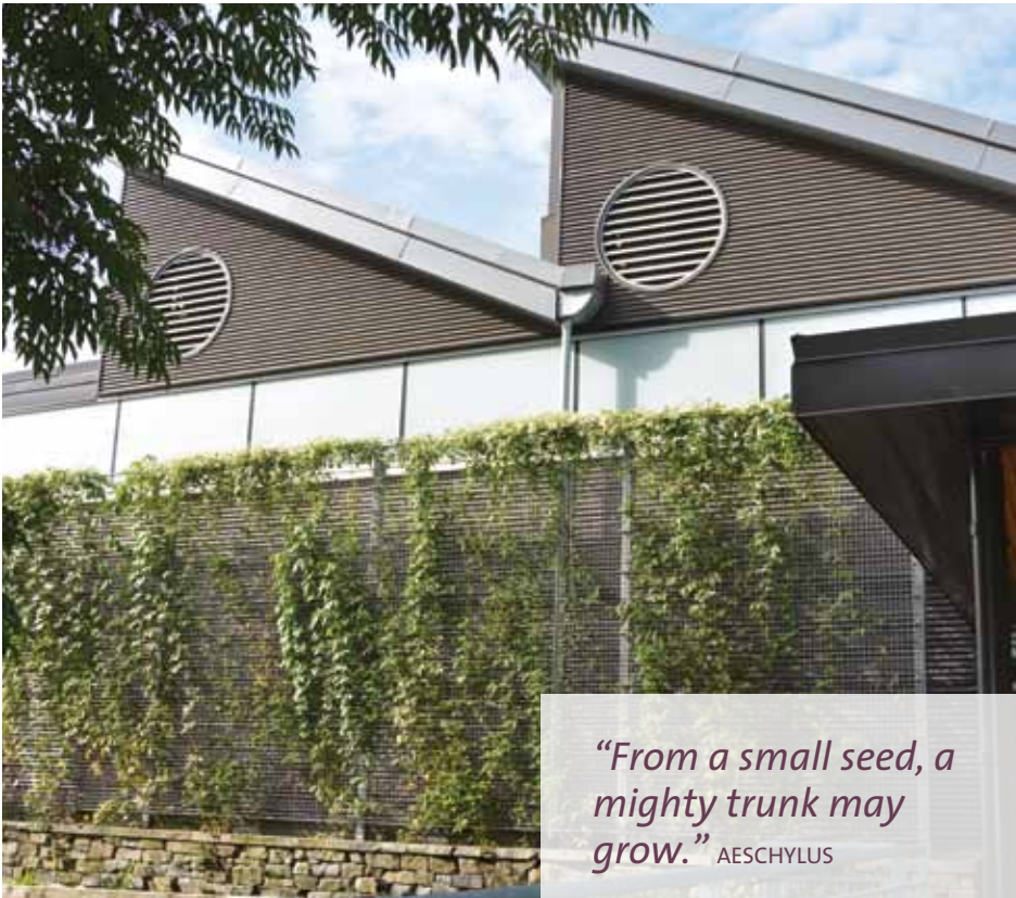
Greenscreen green façade at MEC North Vancouver store designed by Sharp & Diamond Landscape Architecture, supplied and installed by Architek. Image courtesy of Randy Sharp.
