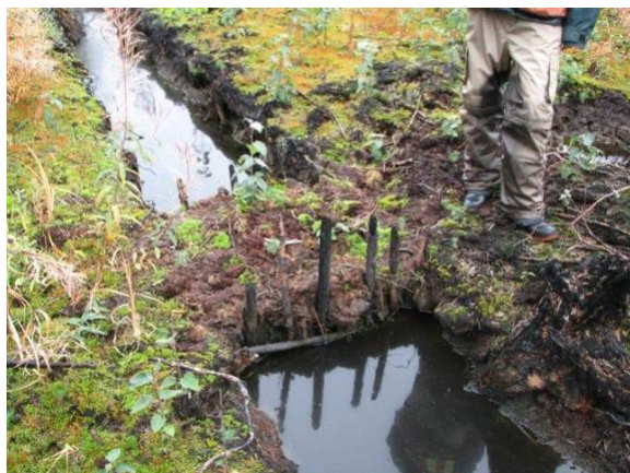
Fig 5. Hand-built dam in a bog ditch, City of Delta, (n.d.)
